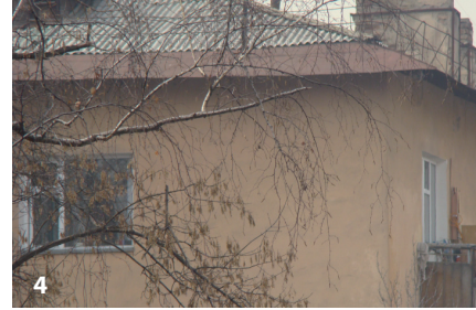
Fig 4. The roof of a residential building in Moscow covered by corrugated asbestos cement sheets.
