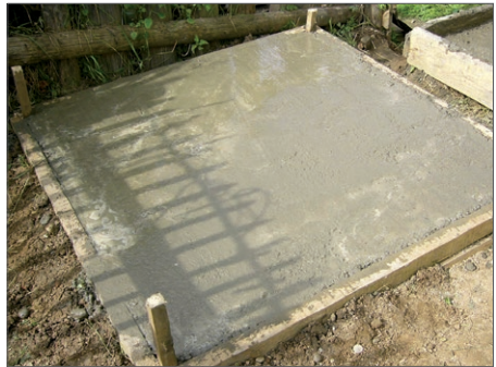
Formwork from wooden slats filled to top with concrete
