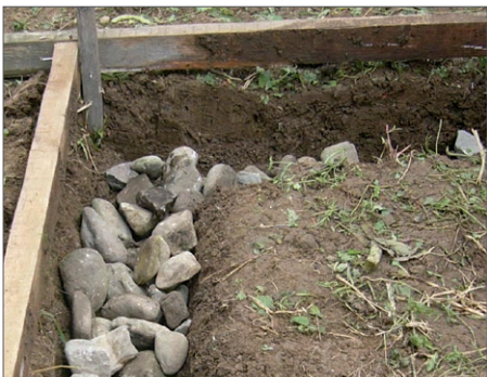
Filling foundation with stones
