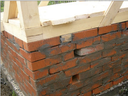
50 mm diameter holes for urine and greywater pipes
