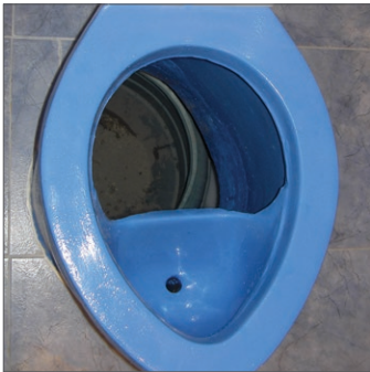
Concrete toilet constructed from a mould
