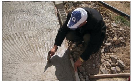
Laying floor slab with high quality concrete
