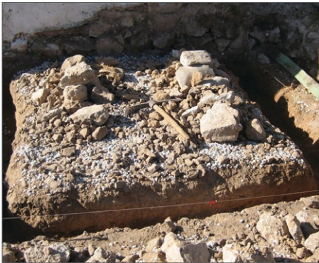
Finished excavated foundation
