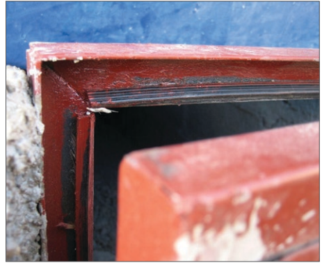
Sealing a vault door with rubber to promote air-tight conditions. Photo from Lukas Ulrich.
