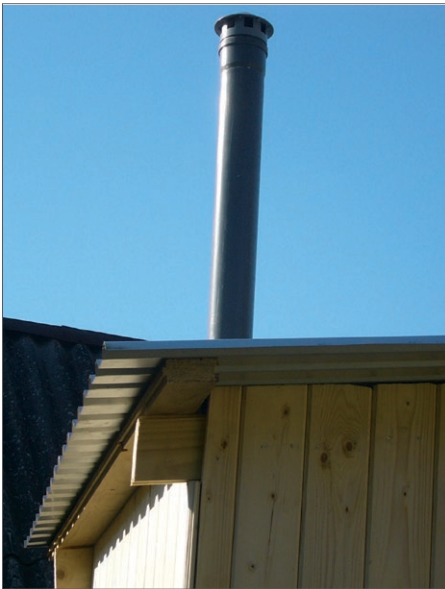
Roof-covering with zinc-covered metal-sheet
