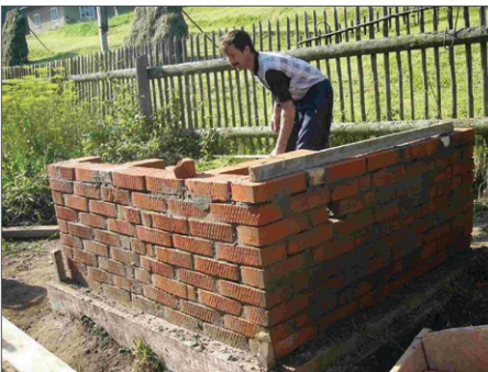
Building dividing wall with bricks
