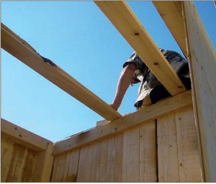
Constructing roof with wooden slats
