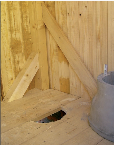
Cutting hole for UD-toilet seat riser into the floor
