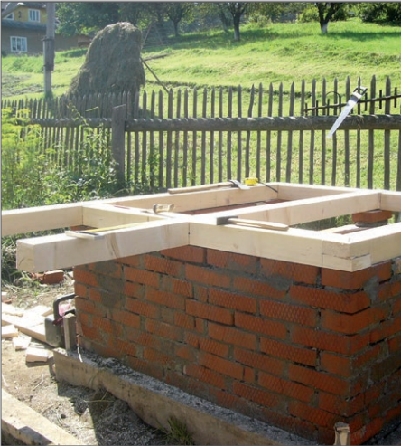
Frame for toilet room floor located on top of the faeces vaults
