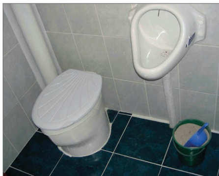
Example of urinal in toilet room
