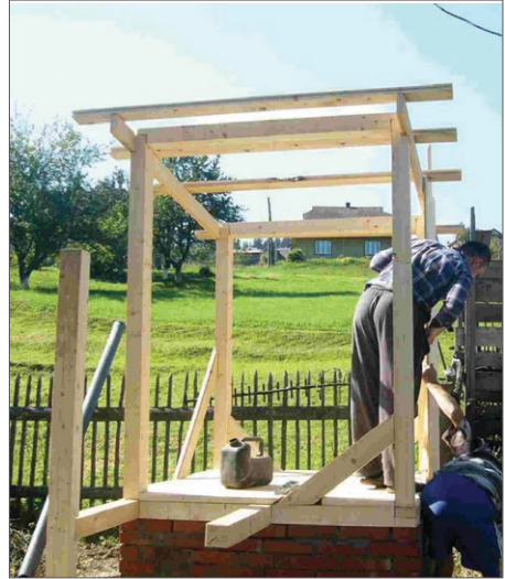
Constructing a frame
