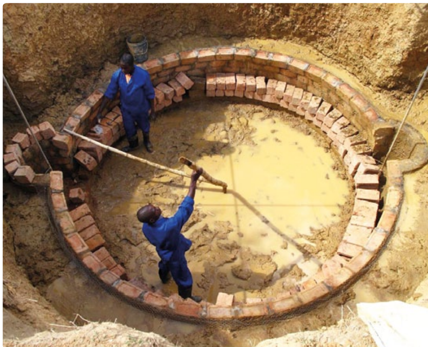
Top left: Construction of fixed-dome biogas plant. Top right: Irrigation of the plants on the newly built constructed wetland, that treats the effluent from the biogas plant. Below right: Peter and Christopher enjoying freshly cooked tea.
