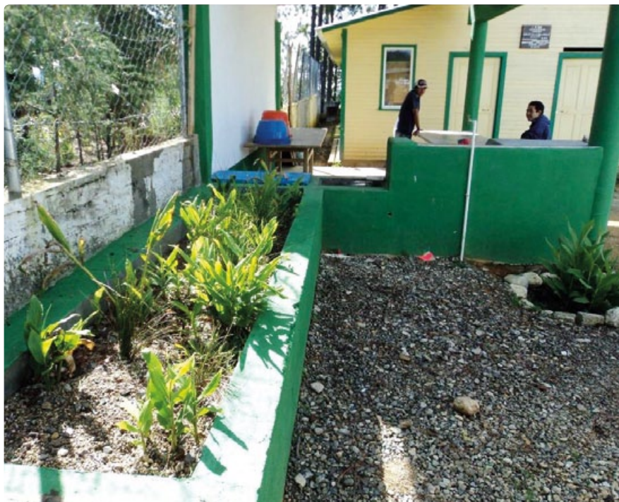
Top left: Local dishwashing practices were considered for the design and construction of this greywater treatment station which begins with solid & grease traps; main treatment is in saturated biofilter, which discharges for irrigation reuse into existing school garden. Top right: SARAR participatory methodology workshops allow for active involvement of the school communities. Below right: A robust concrete handwashing facility was installed at proper height for small users, located just beside existing kitchen. Hygiene & handwashing workshops reinforce behavior change.
