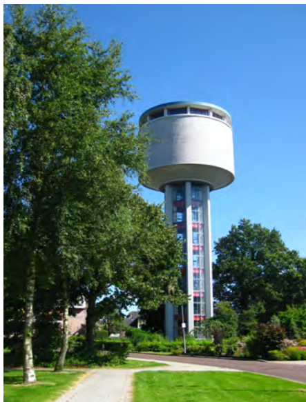
A water tower maintaining an appropriate pressure day and night
