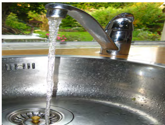
After passing kilometres of pipes, the water quality at household level could be decreased and is often not known.
