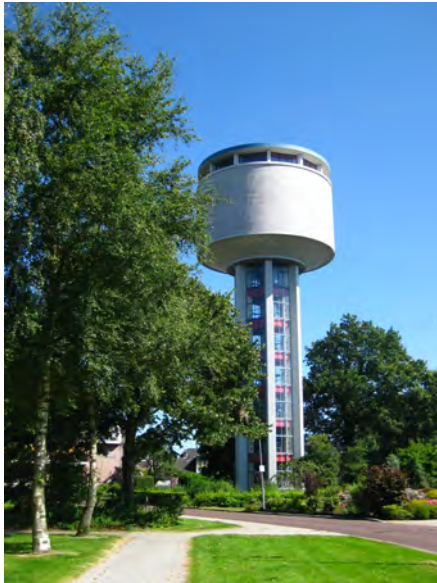
A water tower maintaining an appropriate pressure day and night
