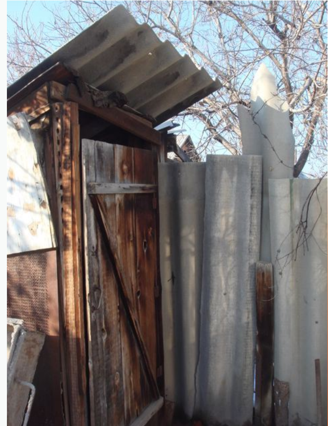
Common sight in EECCA: asbestos slates used in home and garden www.wecf.eu
