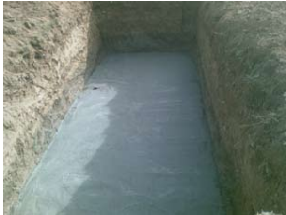
Digging for the settling tank with levelling layer
