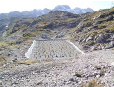
Constructed wetland for greywater treatment in Vorarlberg, Austria
