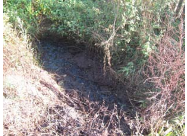
Effluent of the old septic tanks in a gully
