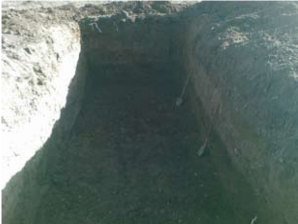
Digging for the settling tank
