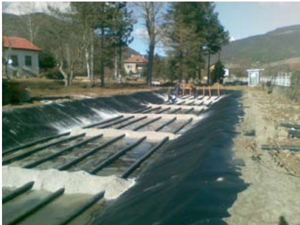
Drainage pipes
