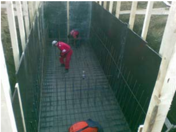
Reinforcement of concrete (settling tanks)
