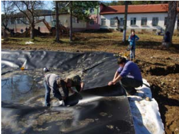
Welding the liner
