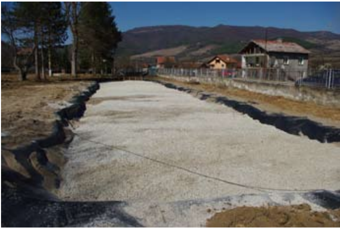
Completed constructed wetland, without plants
