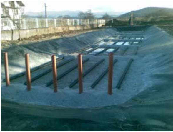
Drainage layer with pipes
