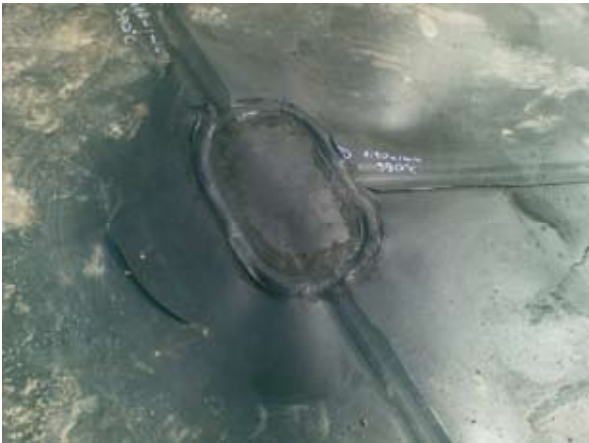
Welding the liner
