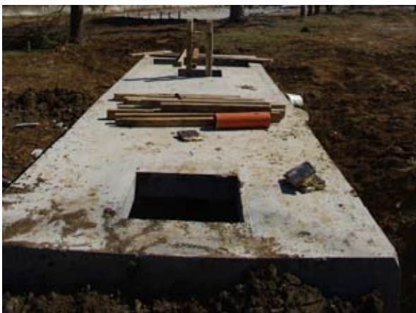
Settling tanks completed
