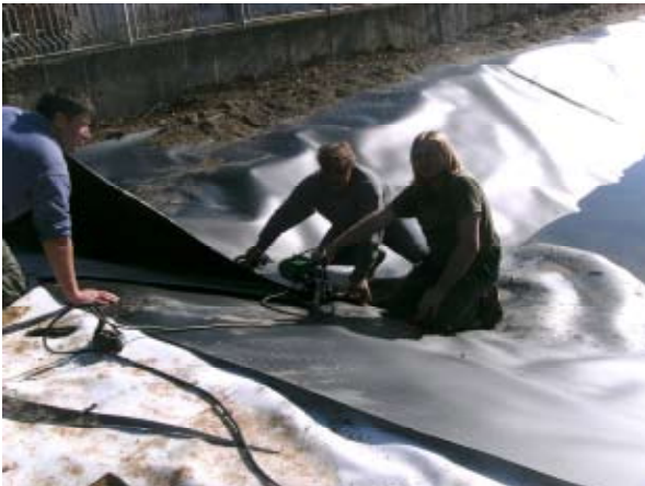
Welding the liner
