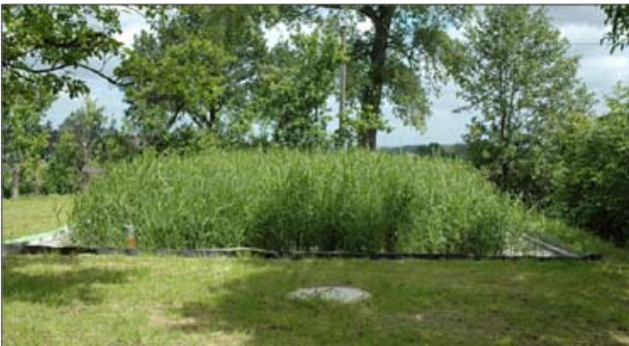
Constructed wetland for municipal wastewater in Örlinghausen, Germany
