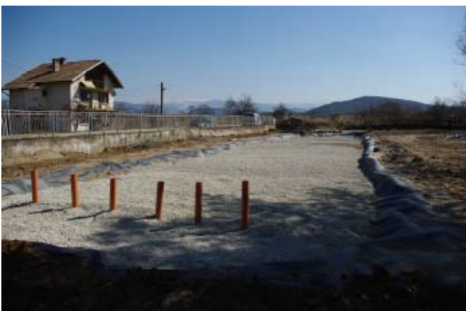
Completed constructed wetland with vent pipes in front
