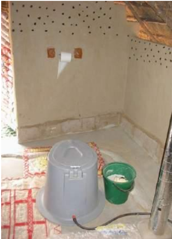
urine diversion toilet made out of plastic
