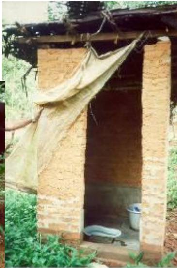
Cemented floor & lower walls
