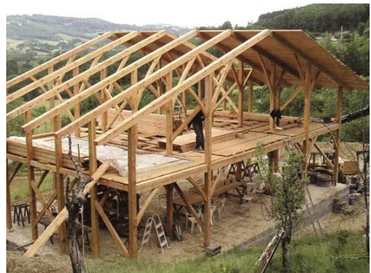
Picture 3: an example of a wooden framework to be filled with straw
