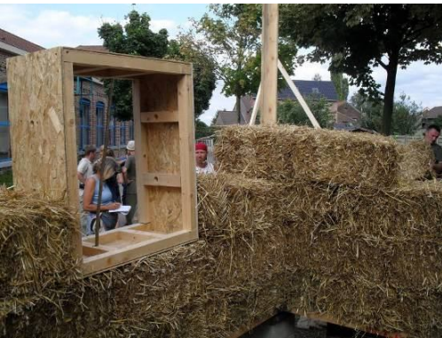
Picture 1 Straw bales are filled into a wooden frame
