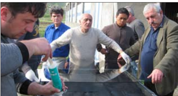
Step 13. Cover the frame with 4 mm thick glass using silicon glue
