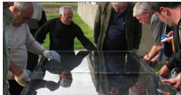
Step 13. Cover the frame with 4 mm thick glass using silicon glue
