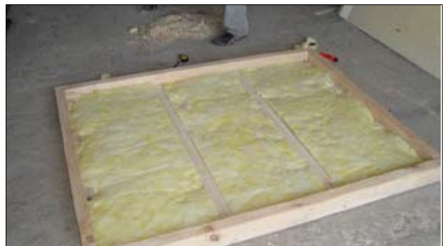
Step 4. Install insulation
