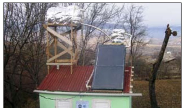
Step 8. Fill collector with anti-freeze liquid
