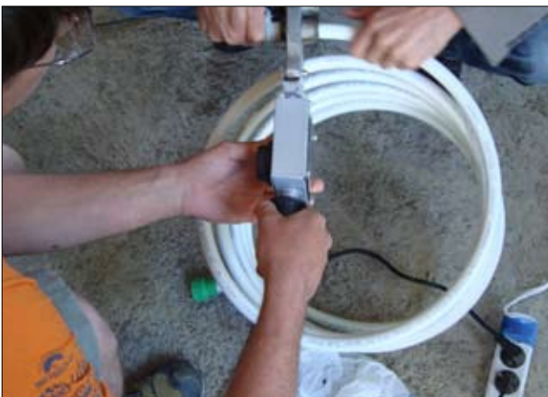
Step 2. Adjust the adapters at both ends of the serpentine
