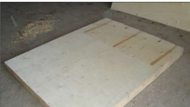
Step 3. Cover the bottom frame with plywood
