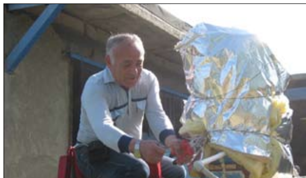
Step 7. Insulate tank and pipes
