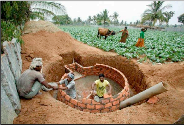
Construction of a Biogas plant in India. (source: Bagepalli Biogas Programme)
