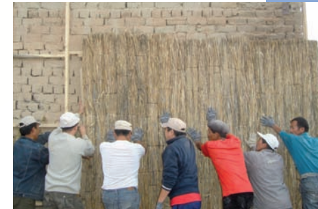
Insulation of wall during a workshop
