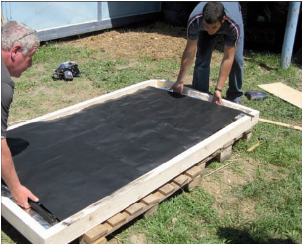
Step 11. Install the absorber into the frame
