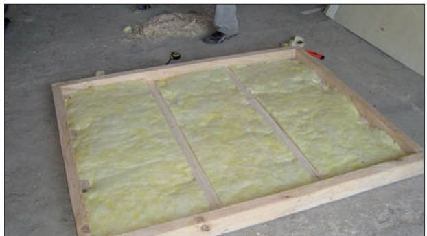
Step 4. Install insulation
