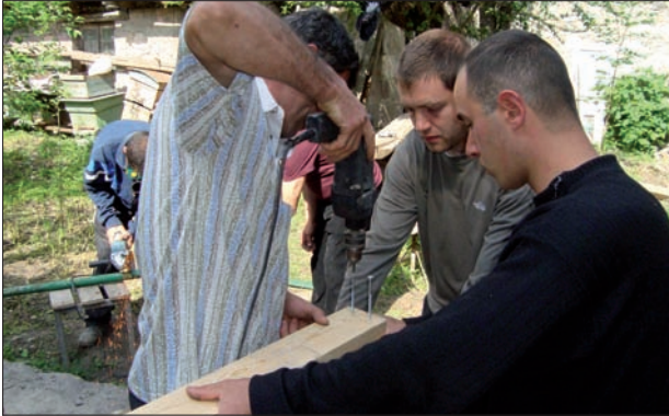
Step 1. Cut framing boards and assemble frame
