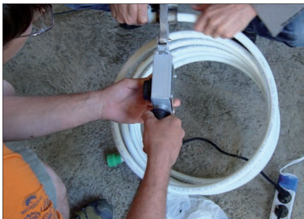
Step 2. Adjust the adapters at both ends of the serpentine
