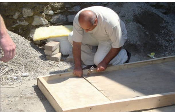
Step 5. Cover the upper part of the frame with plywood, paint black
