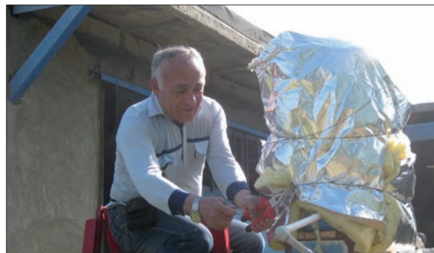
Step 7. Insulate tank and pipes
