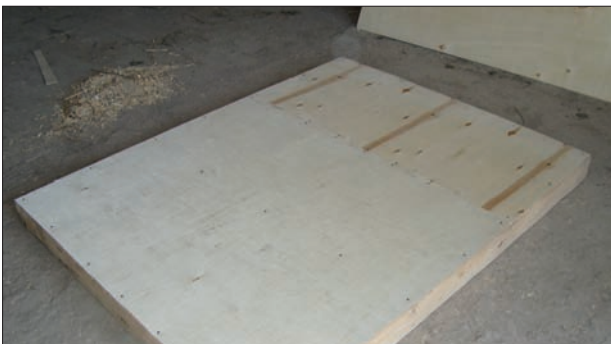
Step 3. Cover the bottom frame with plywood
