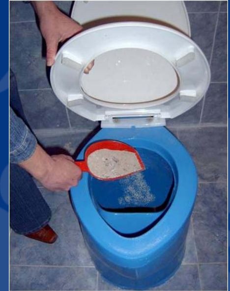
Urine diverting dry toilet
