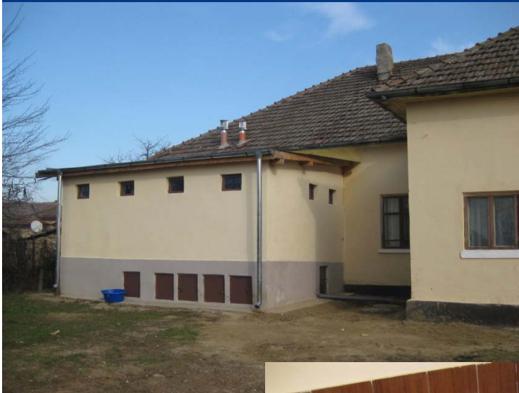
New toilet building attached to the school
