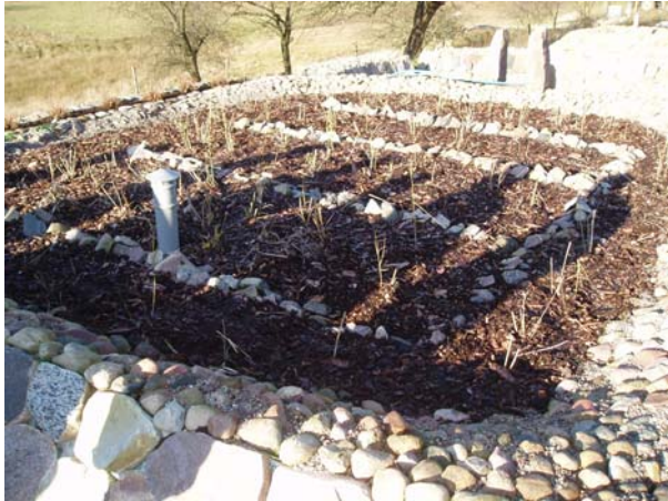
(Constructed Wetland in Poland, Claudia Wendland)
