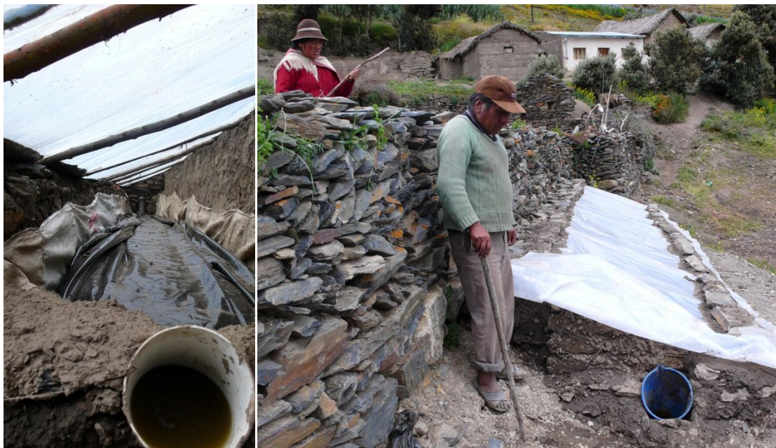
FIGURE 18: TUBULAR PLASTIC BIOGDIGESTER COVERED WITH A PLASTIC SOLAR CANOPY IN BOLVIA (HERRERO 2008)
