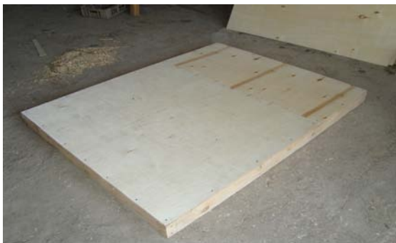
Step 7. Cover the upper part of frame with plywood
