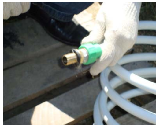
Step 2. Adjust the adapters at both ends of the serpentine
