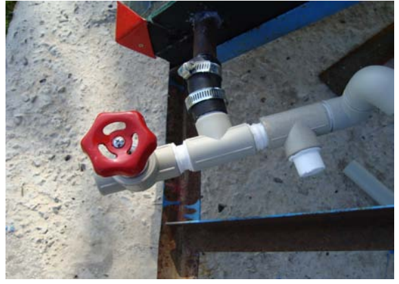
Step 15. Install plumbing outlets and inlets
