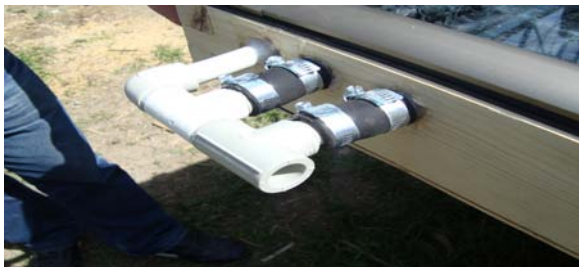
Step 13. Install plumbing outlets and inlets
