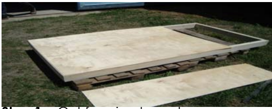
Step 1. Cut framing boards 2. Assemble frame
