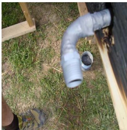
Step 15. Install plumbing outlets and inlets
