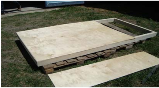
Step 1. Cut framing boards
