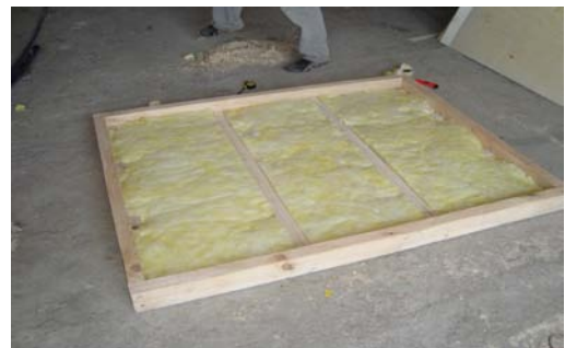
Step 6. Install insulation
