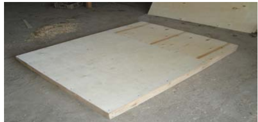
Step 4. Cover the bottom frame with plywood
