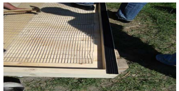
Step 8. Install metal mesh for plastic absorber
