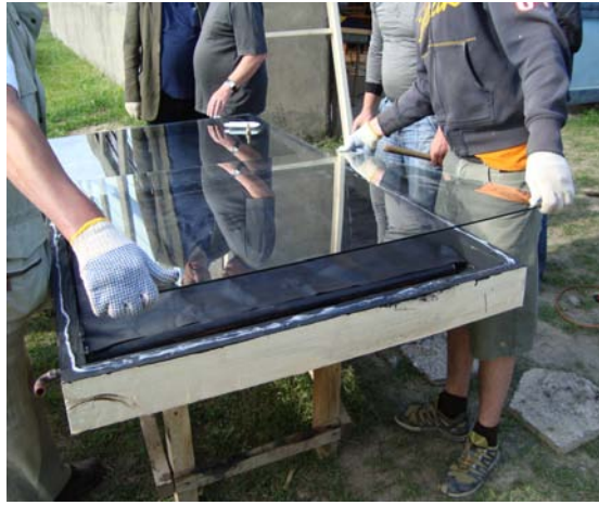
Step 14. Cover the frame with 4 mm thick glass using metal bars or silicon glue
