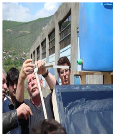
Step 16. Connect the collector to the exchanger in the tank
