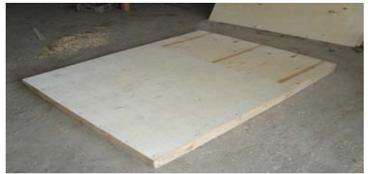
Step 4. Cover the bottom frame with plywood
