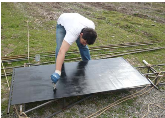
Step 12. Cover with black matt paint or solar lacquer the metal foil and pipes from both sides Step 13. Install the absorber into the frame
