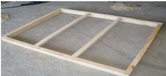
Step 1. Cut framing boards 2. Assemble frame
