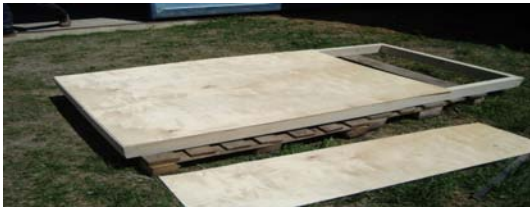
Step 1. Cut framing boards
