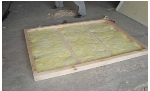
Step 6. Install insulation
