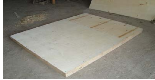
Step 4. Cover the bottom frame with plywood
