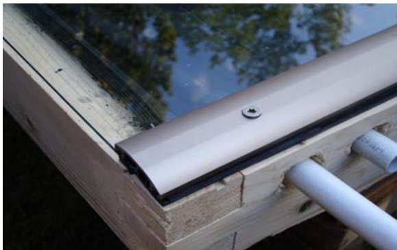
Step 12. Cover the frame with 4 mm thick glass using special metal bars or silicon glue
