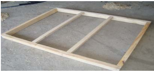
Step 3. Fasten collector bottom and sides
