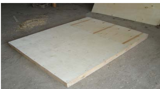
Step 7. Cover the upper part of frame with plywood
