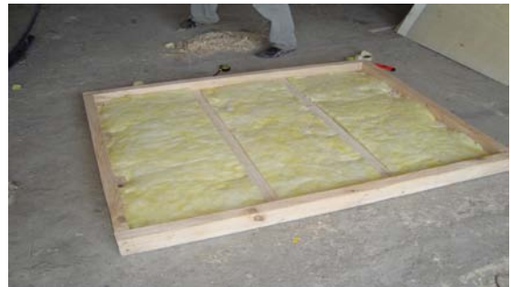
Step 6. Install insulation
