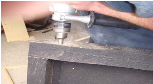
Step 5. Drill inlet, outlet and vent holes
