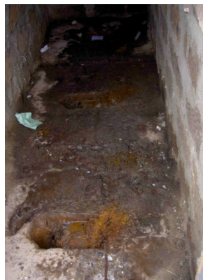
Figure 2. Latrine for 360 pupils: no privacy, unhygienic, cold and slippery during wintertime (source WECF)
