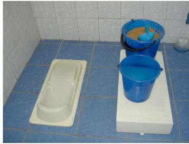
Figure 5. Interior of a double vault dry urine-diverting toilet: Hygienic, safe and easy accessible without leaving the school (source WECF)
