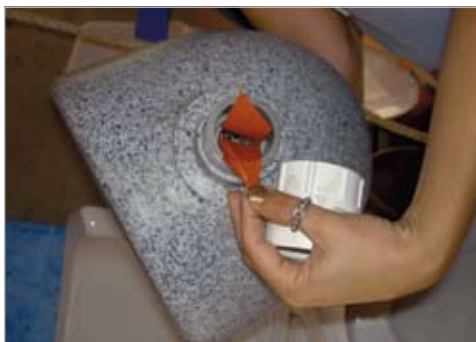
Figure 6: Rubber membrane as odour seal. Photo by WECF
